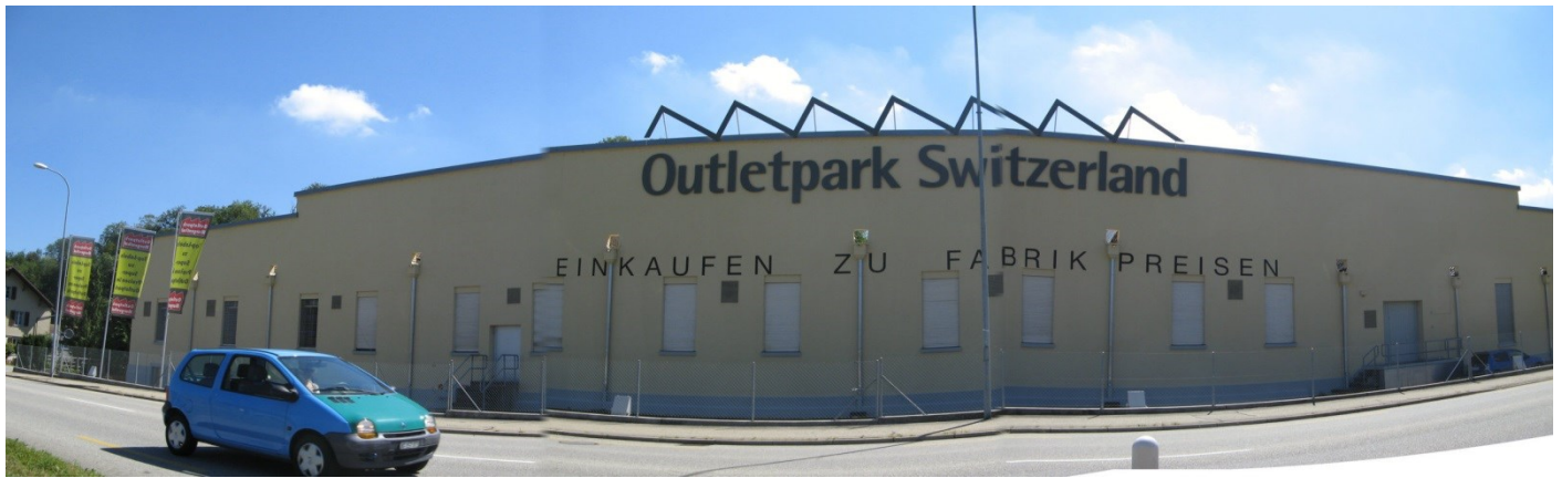
Outletpark Switzerland, Murgenthal (CH) Interdomus AG
