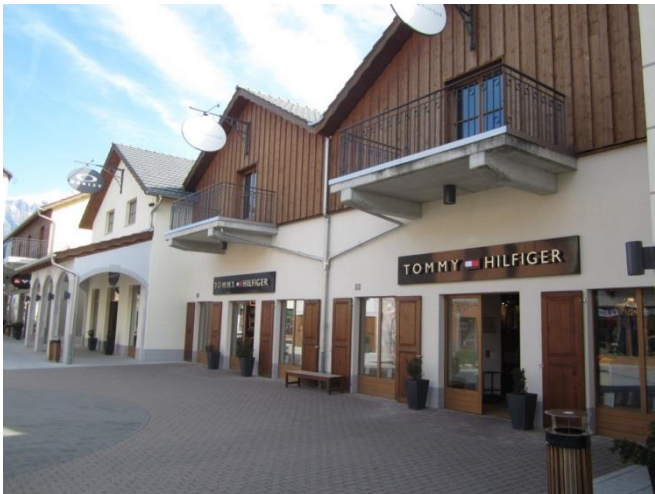
Fashion Outlet Landquart, Landquart (CH) VIA Outlets
